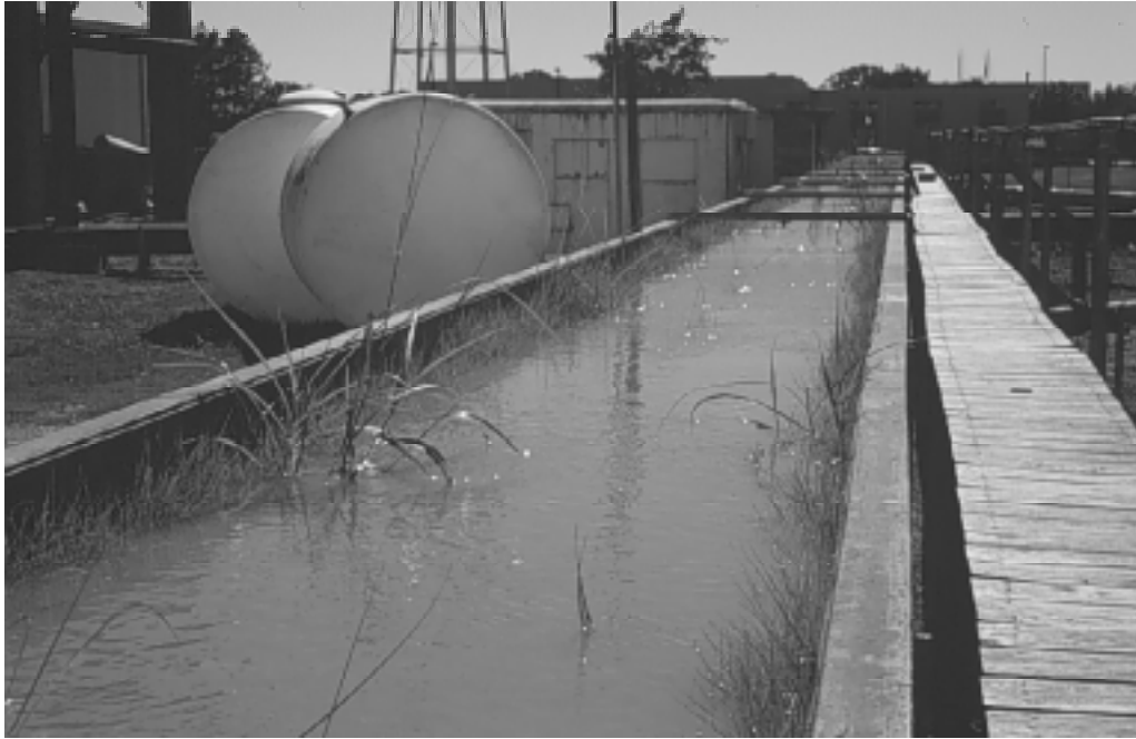
Figure 3.5. Appearance of the swale during an experiment.
