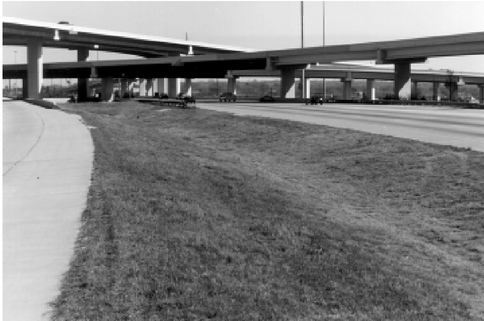
Figure 4.2. Vegetated buffer strip at U.S. 183 site.
