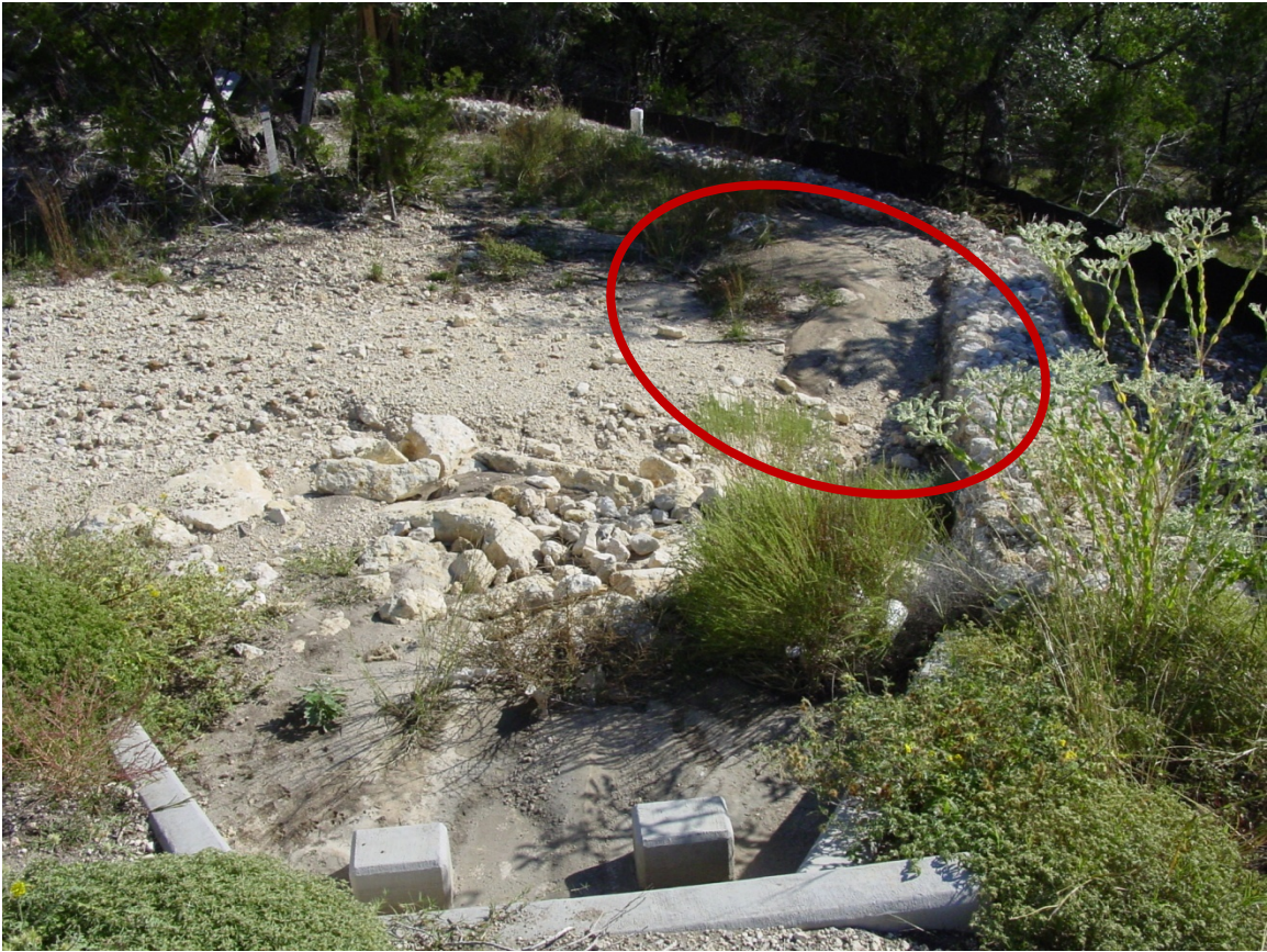
Figure 16: Sediment Accumulation in System V
