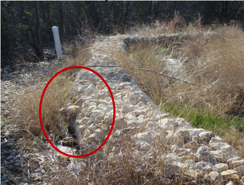
January 2009, Broken Wire Cage
