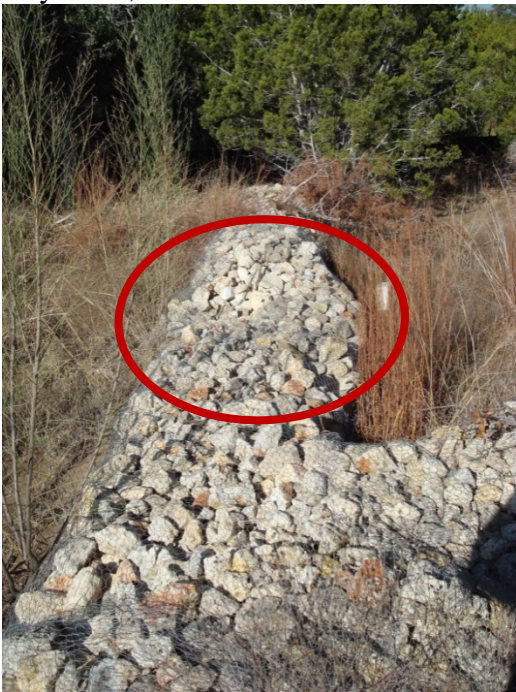
January 2009, Downstream Wire Cage Break
