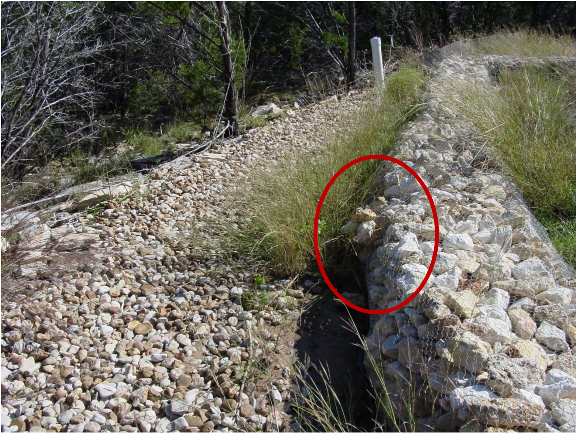
Figure 14: Break in Rock Berm Wiring of System M
