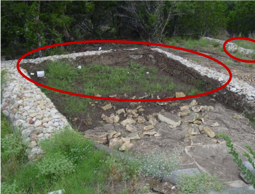
July 2008; Sediment Accumulation and Downstream Cage Break
