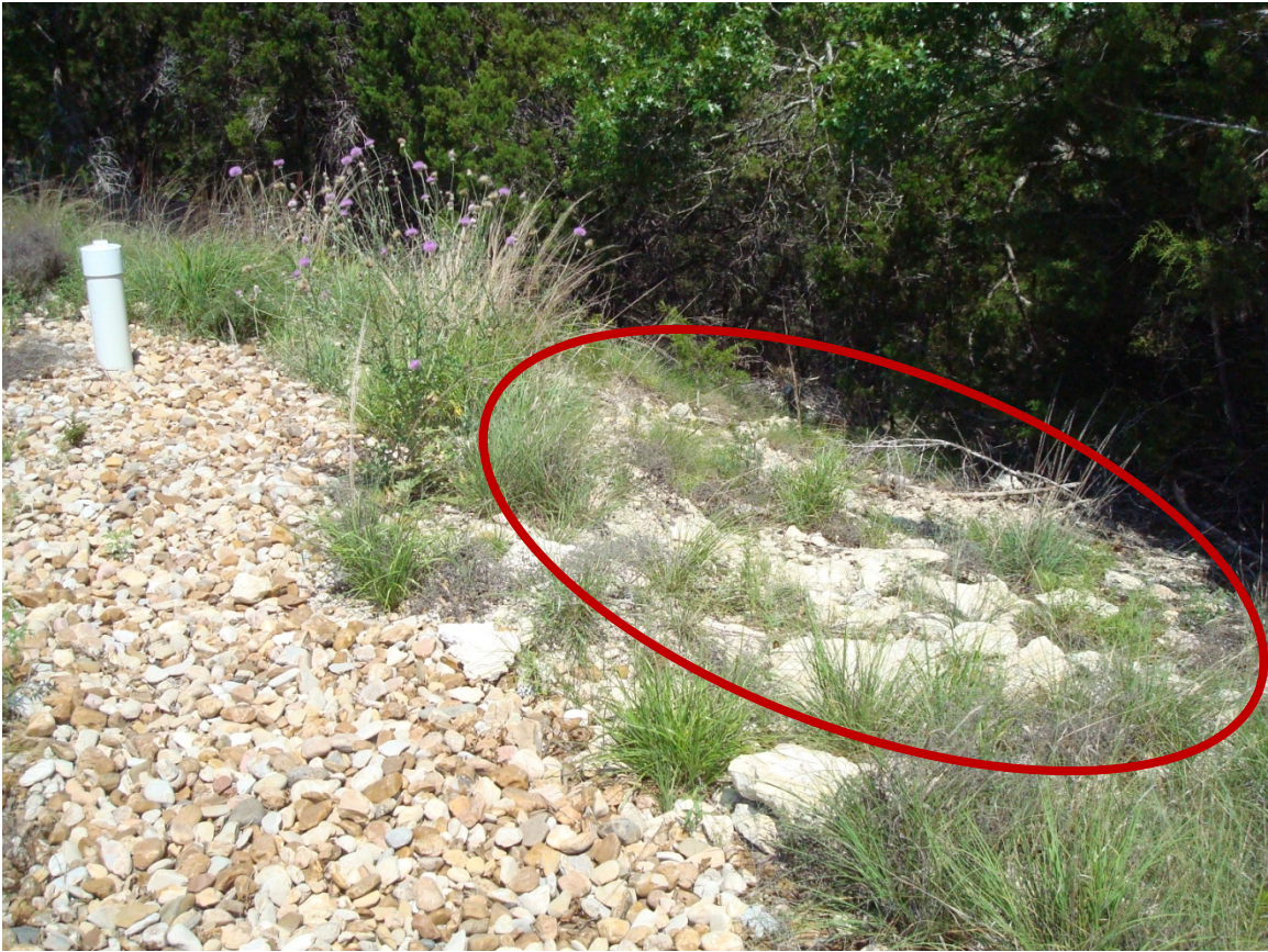
Figure 15: Downslope Erosion on System T
